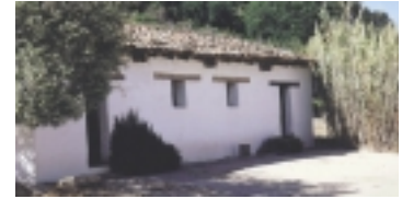
Adobe building, La Purisima Mission, Lompoc
